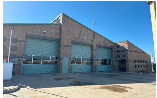
Fire Station 609 at SDL: Airside View
