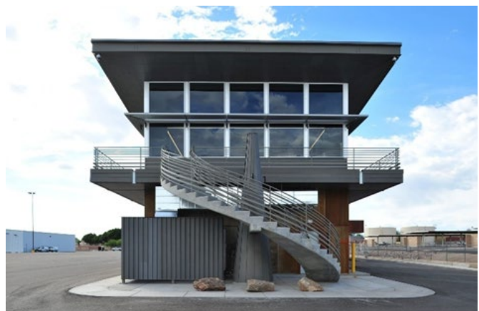
Airport Operations Center Looking West
