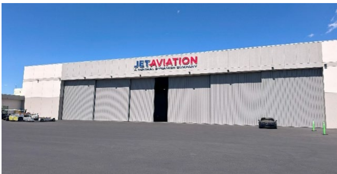
Jet Aviation Hangars
